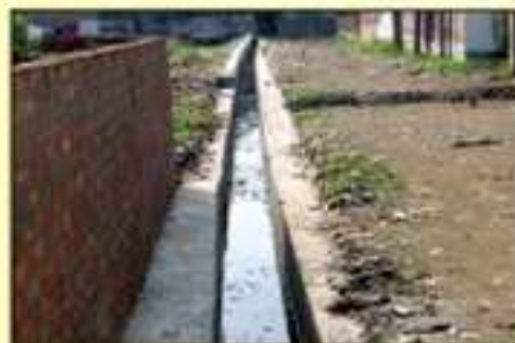
Regradation of Storm water channel at HMC ward No. 50
