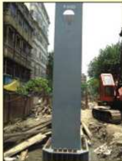
Pier Vivekananda Road Flyover
