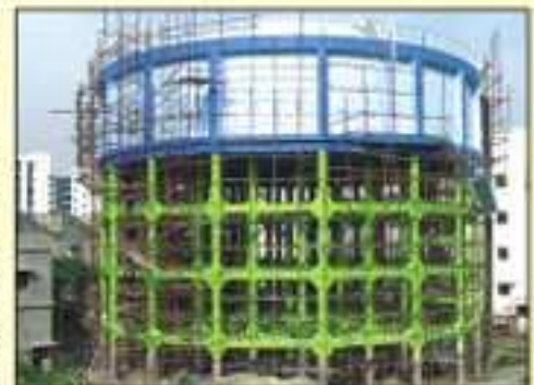
Construction of overhead reservation under water supply for Sector-V, Salt Lake
