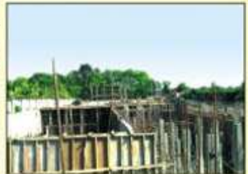
Construction of filter led for 15 MGD Water Treatment Plant at Bansberia
