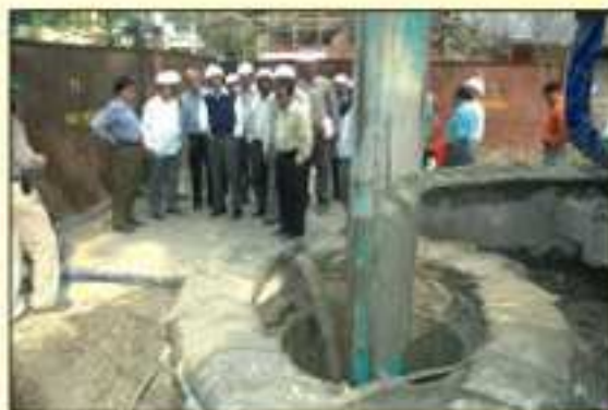
Construction of Vivekananda Road Flyover
