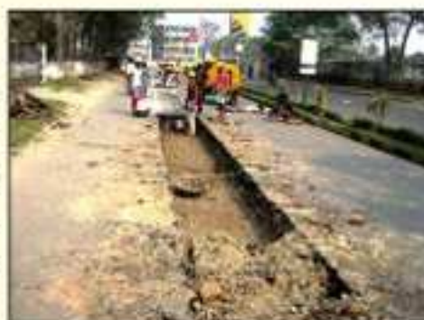
Road digging for sewerage project, Salt Lake, Sector-V
