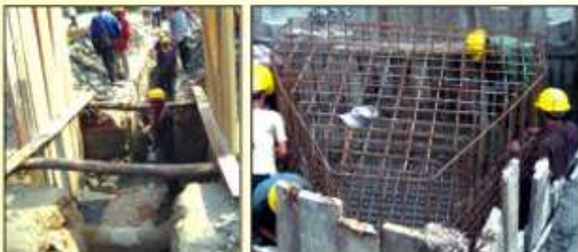
Water Supply & Sewerage Project in Sector - V, Salt Lake
